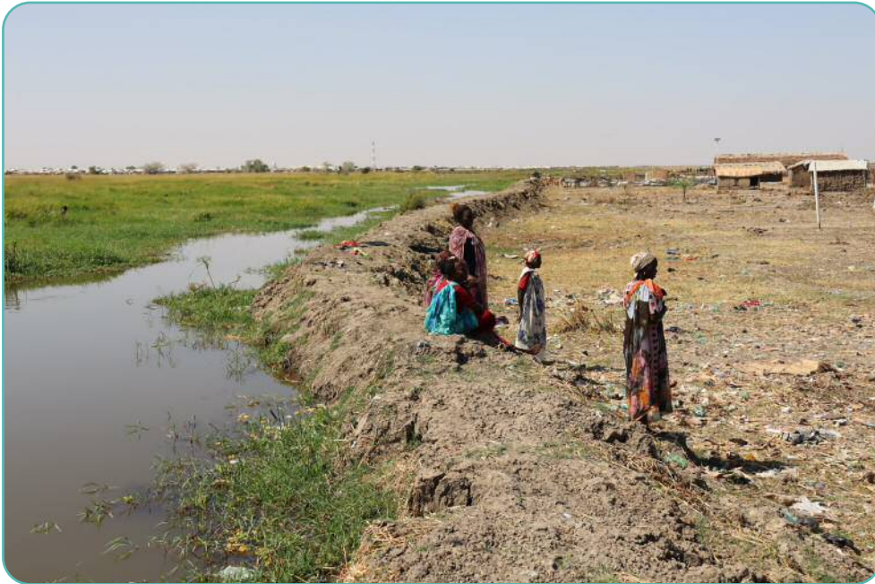
Fig. 04: Example of an earthen dike in the Al-Redis Refugee Settlement. Philippe Reymond, UNHCR 2023.
