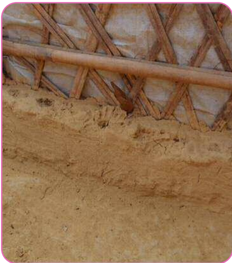
Fig. 13: Structure consolidation through reuse in the refugee camps. E. Cauderay, CRAterre, 2019.
