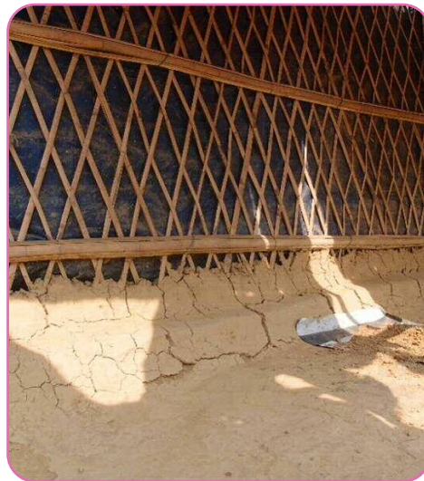
Fig. 12: Structure consolidation through reuse in the refugee camps. E. Cauderay, CRAterre, 2019.
